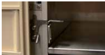
Easy release handle to open master gate
