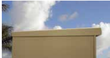
Sloped top for moisture runoff
