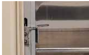
Easy release handle to open master gate
